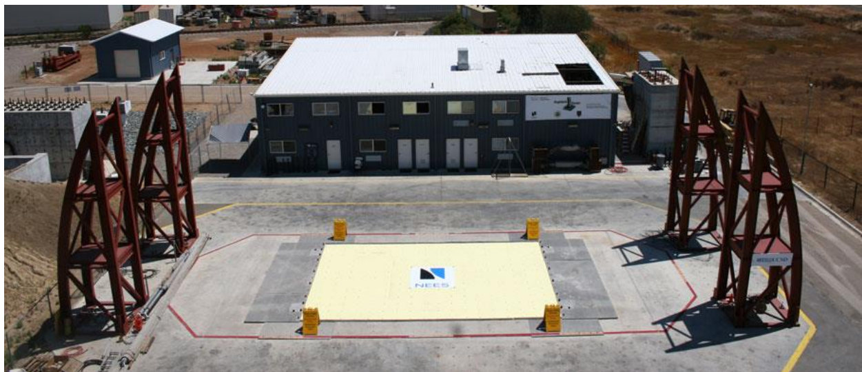
Figure 8.1: University of California San Diego Large Earthquake Shake Table
